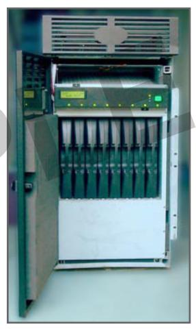
Fuel cell cartridges visible below control panel
